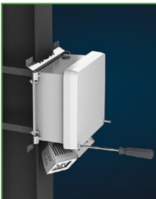
Unscrew access door screws.
