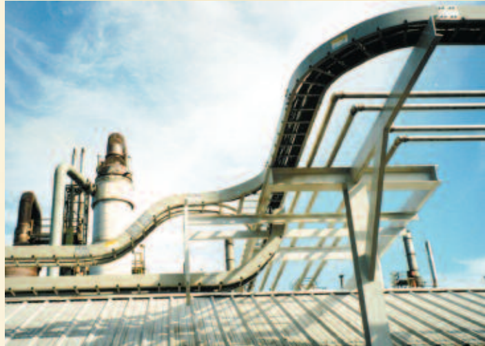
Horizontal and vertical drops, exterior installation.
