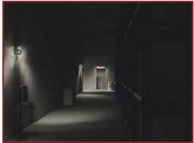
3D image lighting rendering showing installation of two RG-NX Series battery units and a LNC combination unit in an industrial application under emergency lighting conditions.
